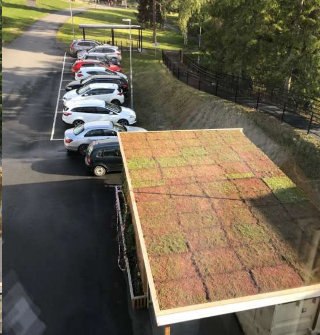
Green roof at Sunnaas newly installed fall, 2018
